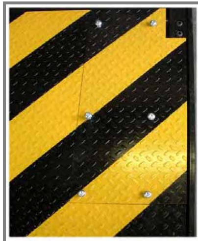
Blocker side inspection plates.
